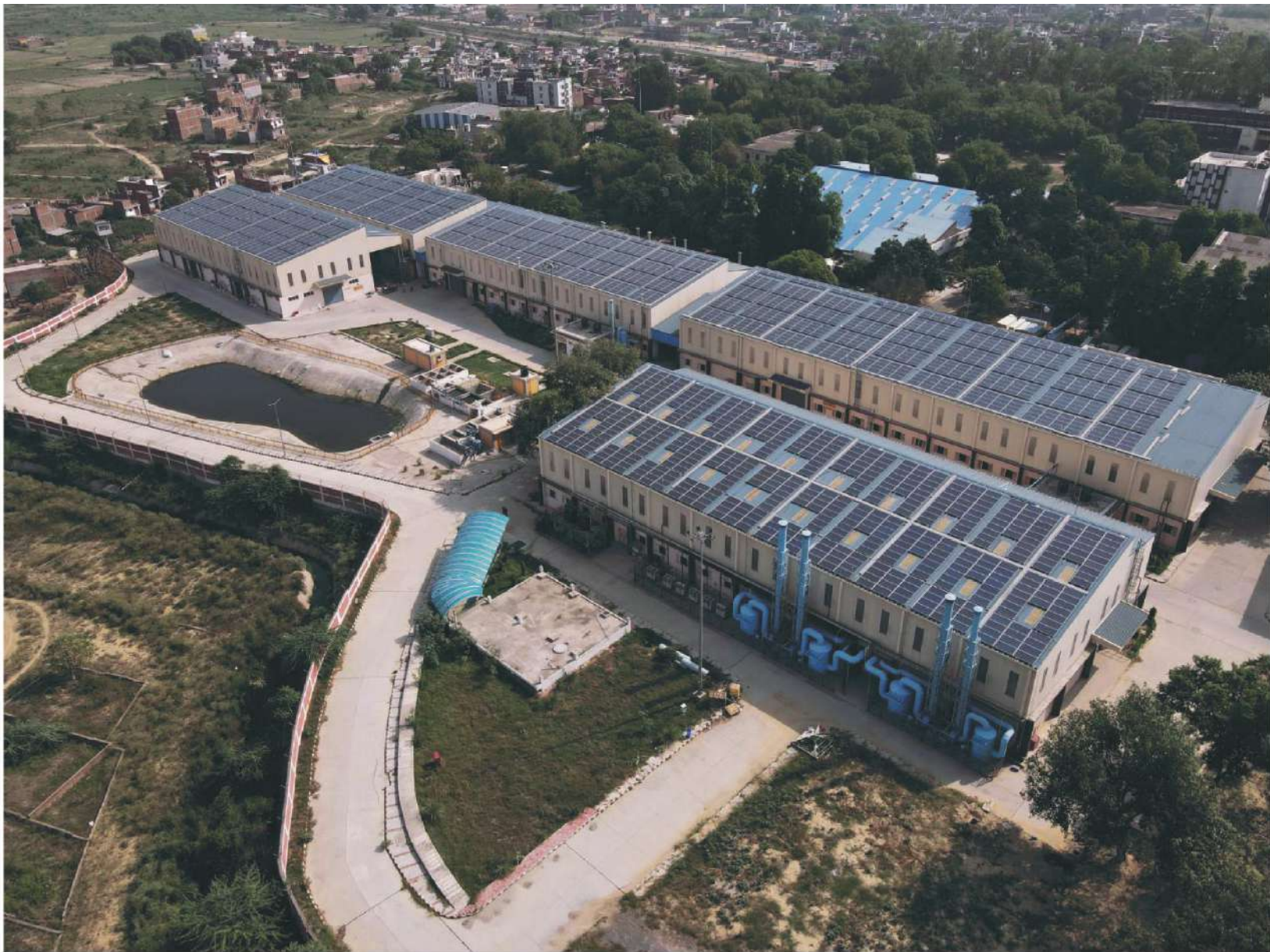
ALIMCO Modernized infrastructure have provision of roof top solar panel system with installed capacity of 1250 KW.
