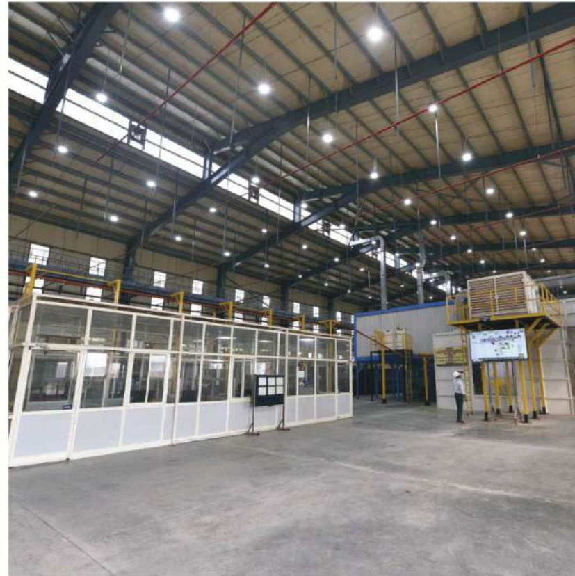
Automated Powder Coating Plant (Work Centre6) :
