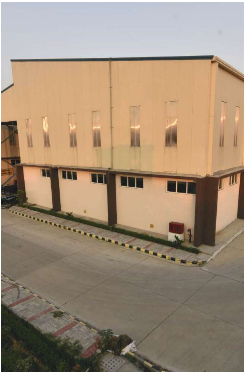
Covered storage with G+2 storage levels for storage of finished goods equipped with goods lift.
